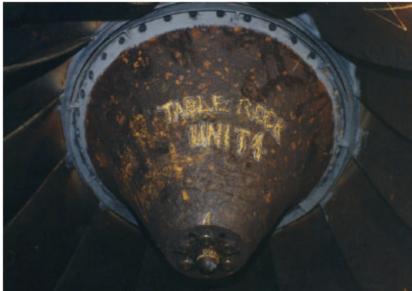
Figure 6. Modifications Made to the Hub on Table Rock Unit 2
