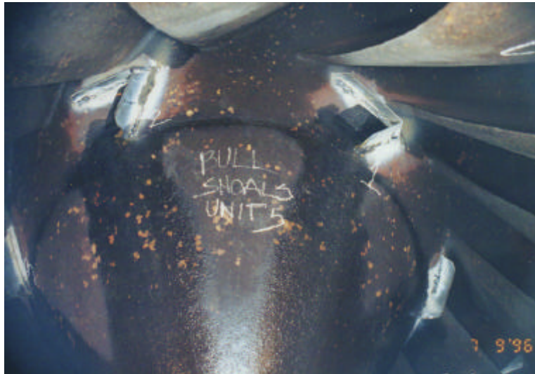
Figure 3. Hub Baffles Installed at Bull Shoals Dam
